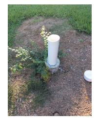
On a properly completed well, the well inspection port should be accessible. It allows access to measure the water level or access to chlorinate the well in the event of a positive bacteria test.
