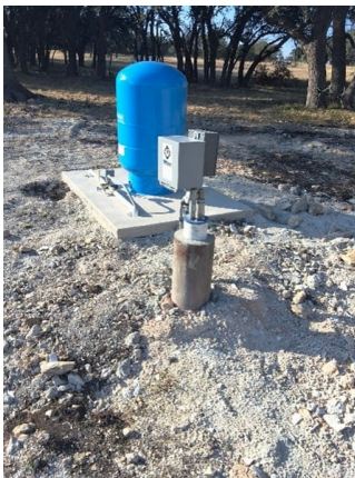
A properly completed well
